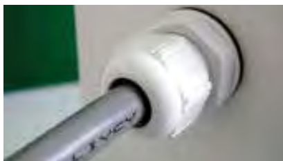
4. Put the cable through.
