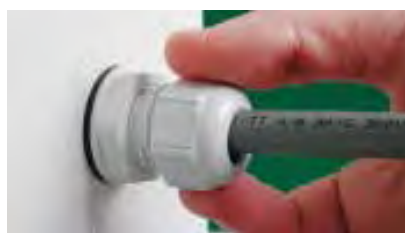
5. Tighten the gland with a clockwise rotation.
