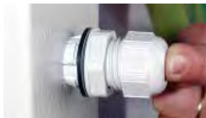
2. Press the gland in to the housing.
